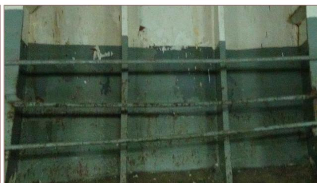
*Bulkhead frame inadequately covered with railings*
